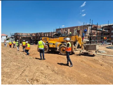
Picture 3: Construction site visit (Riverside).
