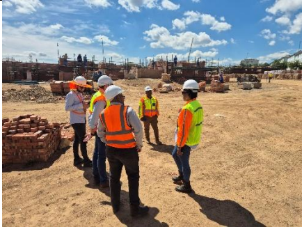
Picture 3: Construction site visit (Riverside).
